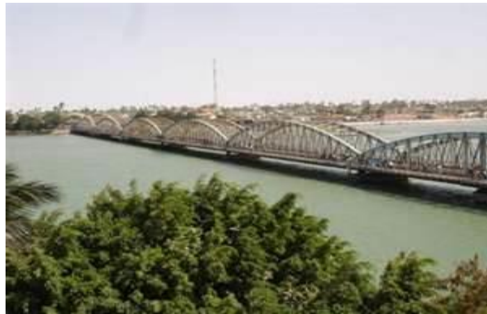
Photograph 1: Faidherbe Bridge, Saint Louis
